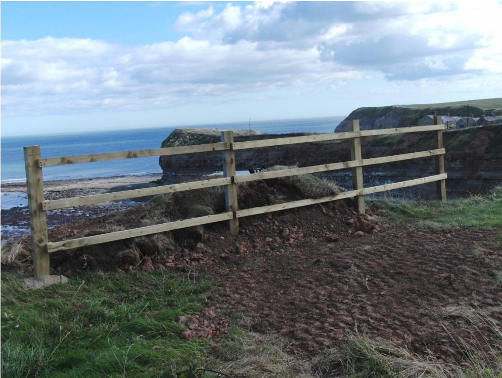
Figure 14 Fencing erected around the scanner housing
