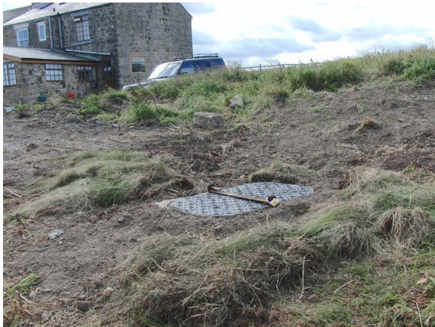
Figure 2 View of the sealed seismometer installation, flush with the ground, and set back from the edge of the cliff by 5 m.
